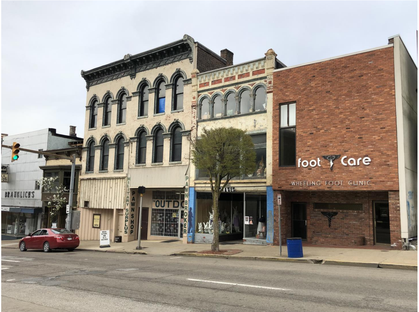
Photo 6. 1061-1073 Main Street, facing southwest
