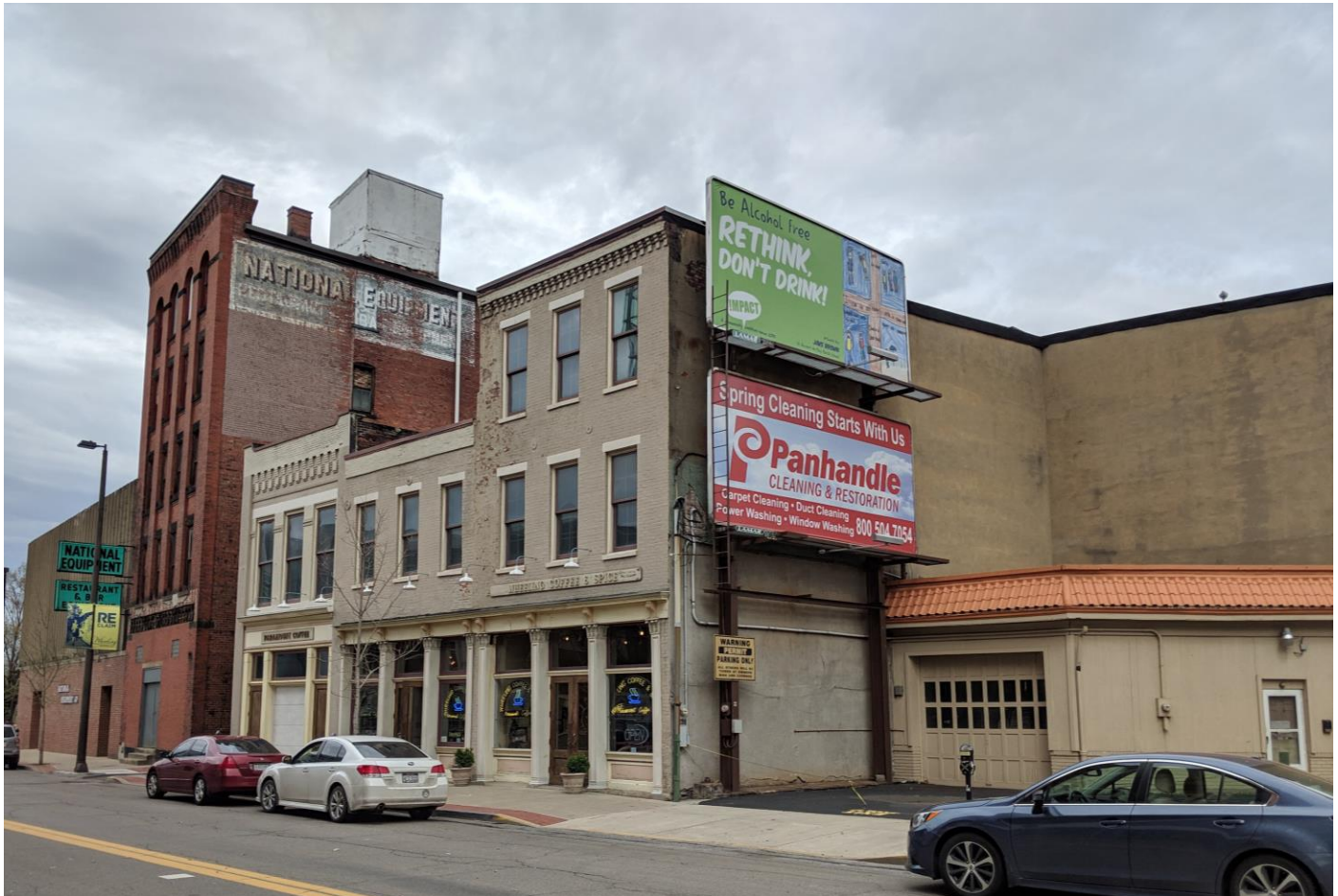
Photo 12. 14th Street at Main, facing northwest
