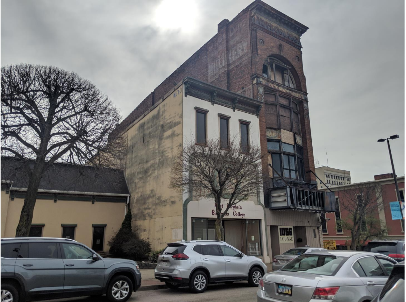
Photo 5. 1052-1056 Main Street, facing southeast
