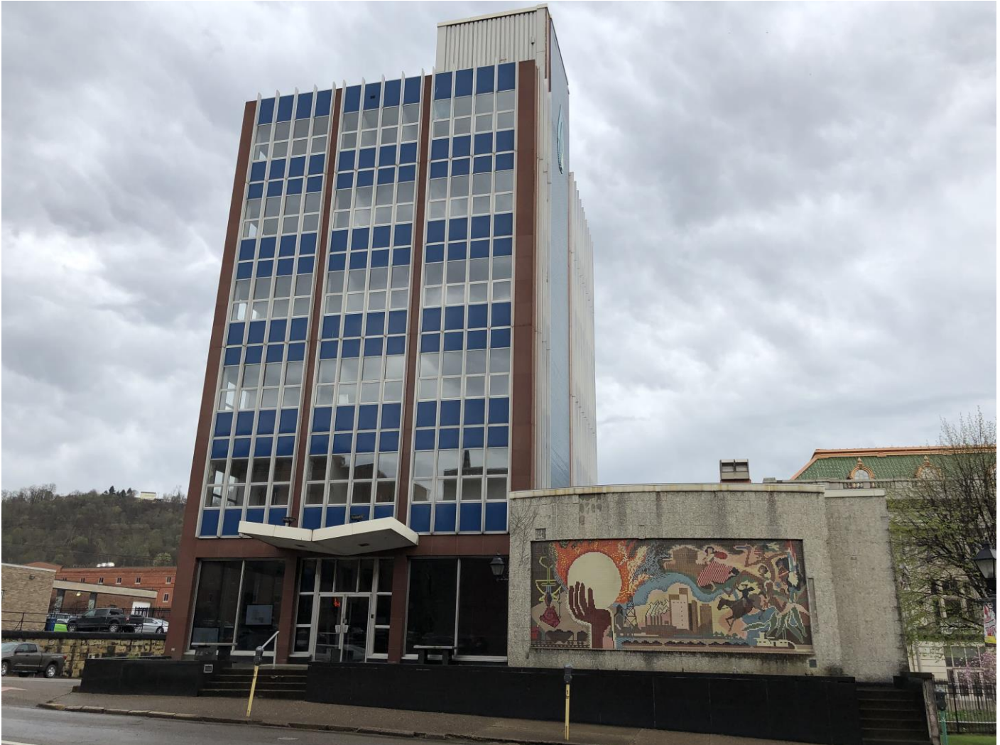
Photo 17. Columbia Gas of West Virginia Building, facing south
