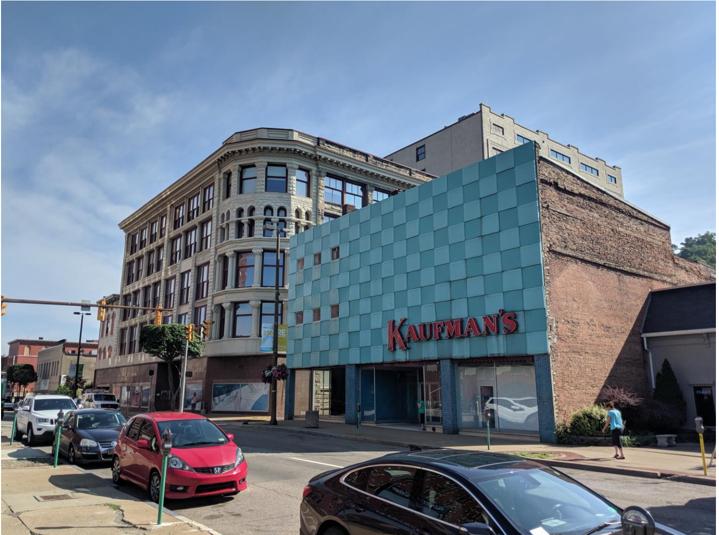
Photo 4. Main Street south of Lane 7 Alley, facing northeast
