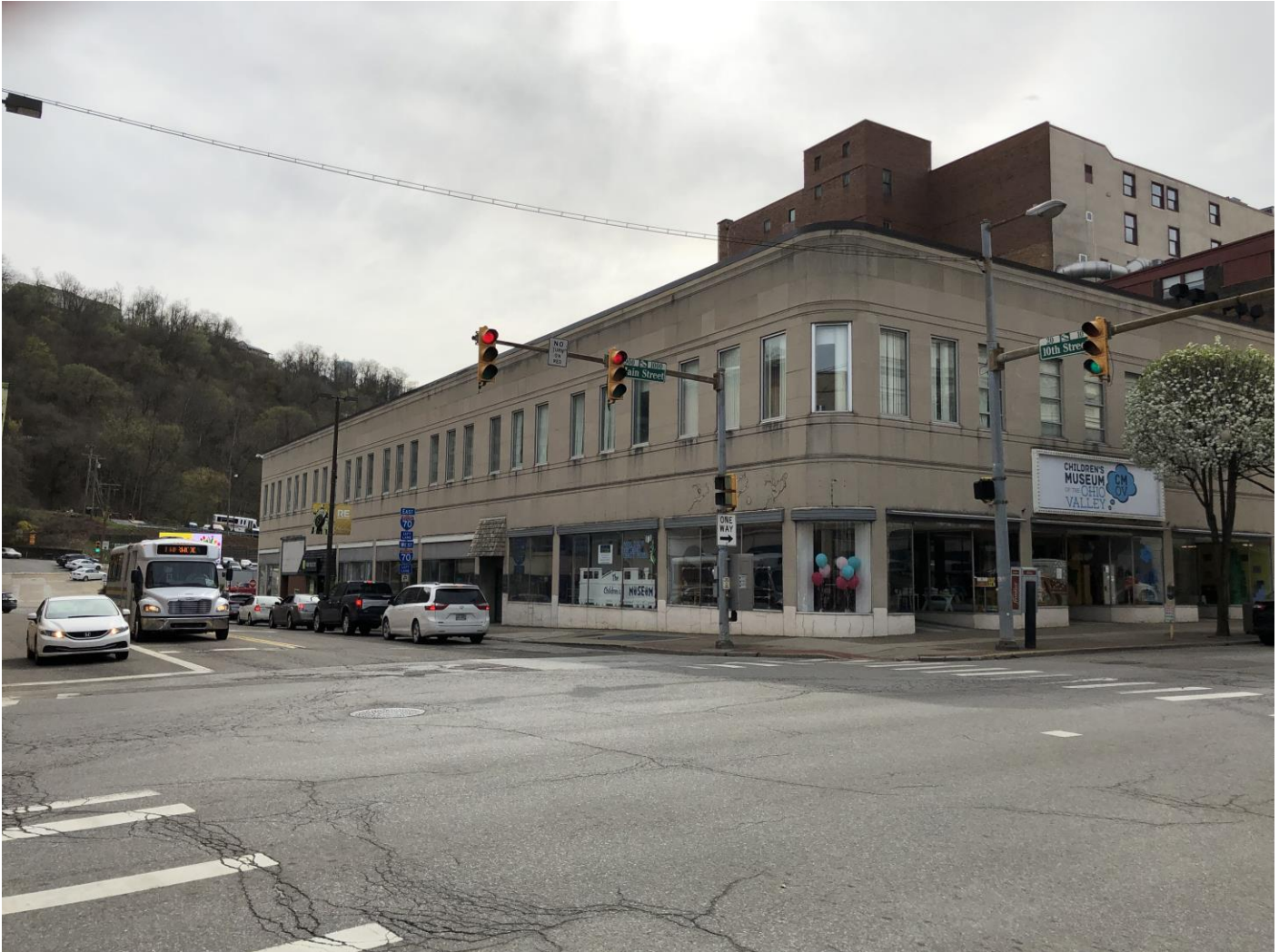
Photo 3. Main and 10th Streets, facing southeast
